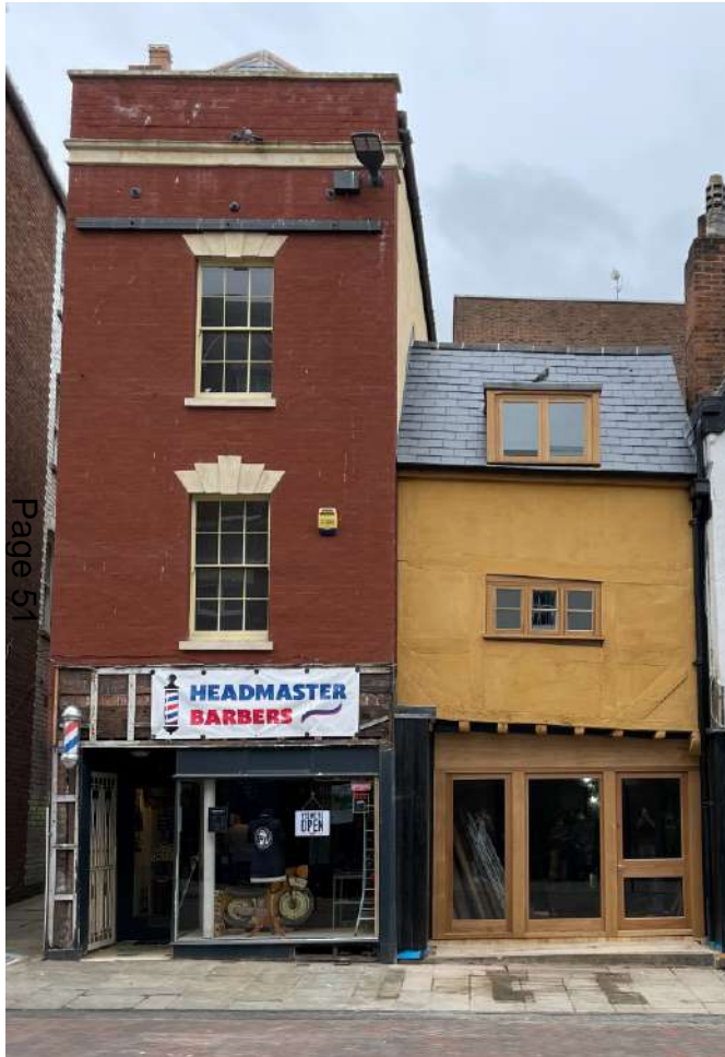
Sixteenth-century timber framing (right) and nineteenth-century brick façade (left) at 39-41 Westgate Street—both Grade II listed buildings. Photo: GCC.
