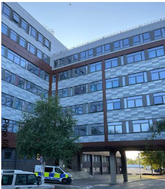
The Shire Hall extension. Photo: GCC.
