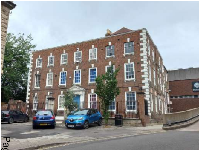
Winston Hall, Constitution Walk (Grade II* listed). Photo: GCC.
