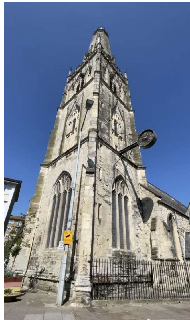
St Nicholas's Church, Westgate Street. Photo: GCC.
