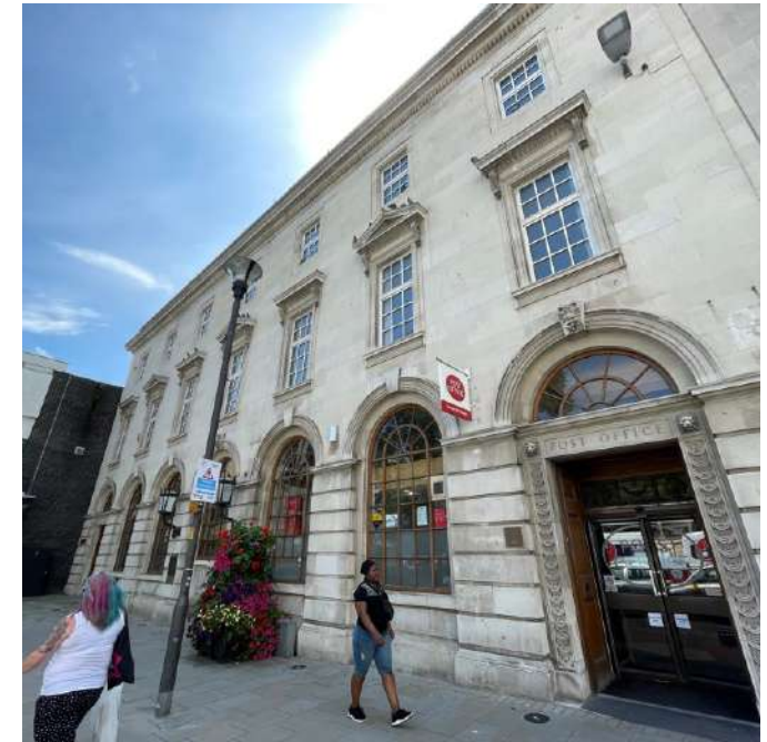
The Post Office, Oxbode. Photo: GCC.
