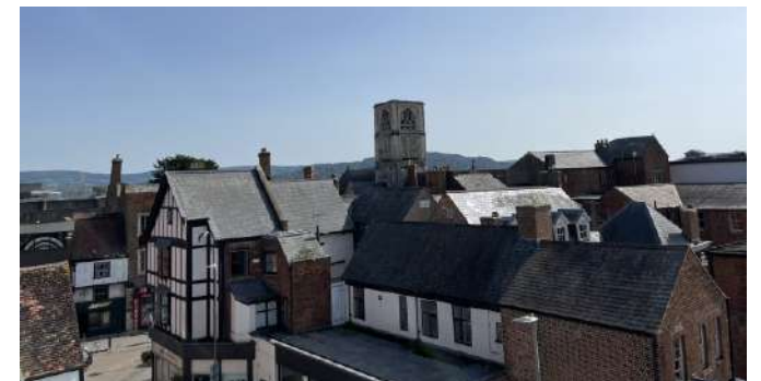
Looking south from Longsmith St carpark. Photo: GCC.
