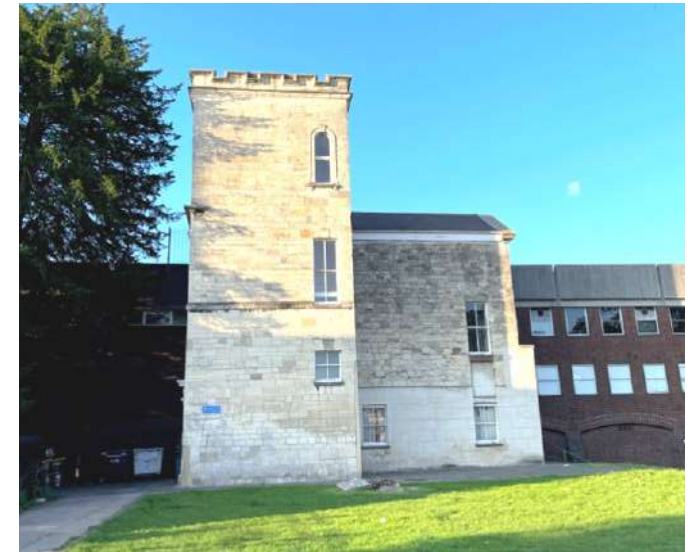
Addison's Folly (Grade II listed) with the Eastgate Shopping Centre visible behind. Photo: GCC.
