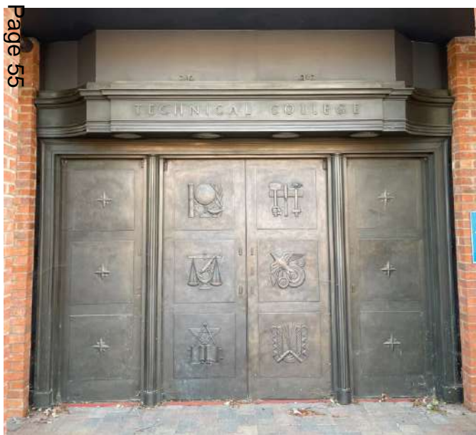
The cast bronze doors of the now demolished Technical College, preserved as part of the Friars Orchard development. Photo: GCC.
