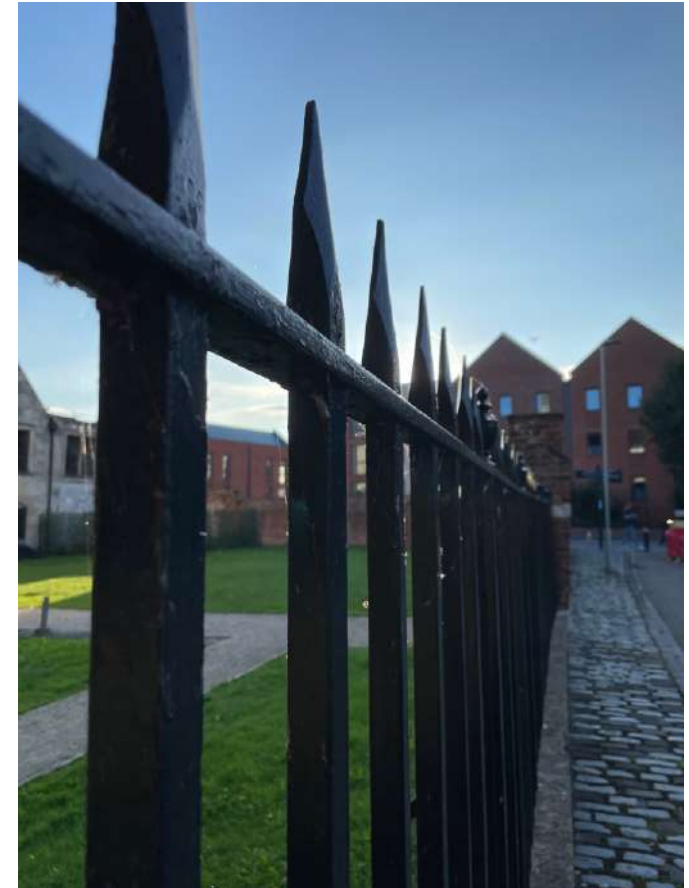
Boundary railings at Blackfriars. Photo: GCC.
